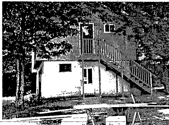
Boy's Dormitory - 1999 A second story was built on top of an original dorm to accommodate additional campers.
