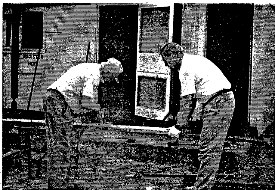
Rev. Bill Hossler, District Superintendent 1998 - Present Mr. Wilbert Steele (left) working with Rev. Bill Hossler on the Camp Office renovations.
