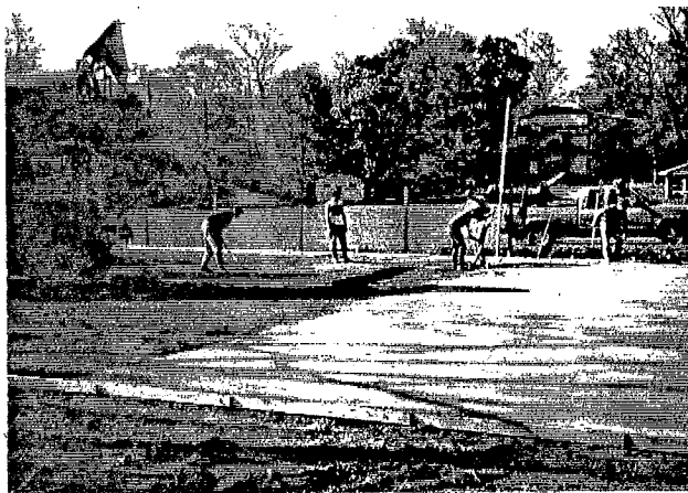
Making of the Basketball Court - 1998 Men from our Wilmore, KY church help to pour the court.
