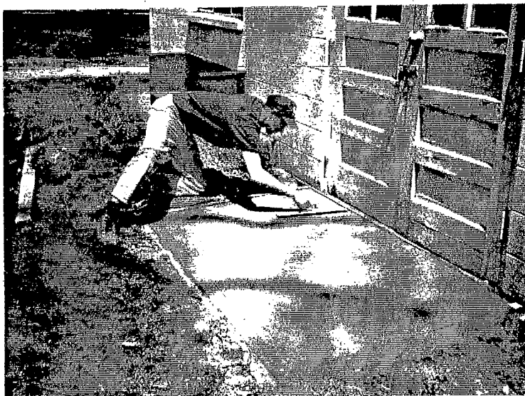
Dale Beyer putting the finishing touches on the newly poured walkway into the children's tabernacle.
